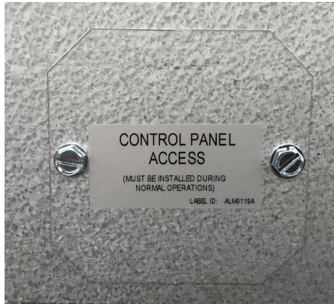
Figure 1 – Control Board Access
